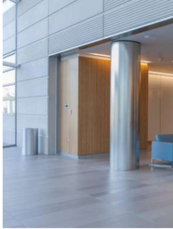
Stainless steel Column Cladding
